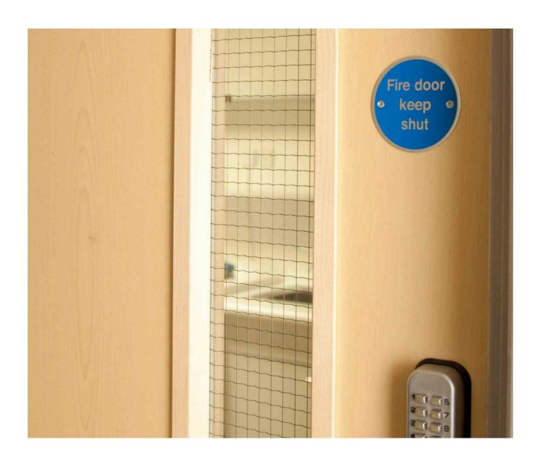
Door Leaves in excess of 450mm wide must contain a vision panel to meet Doc M and BS8300 standards. Vision panels may be reduced / omitted on internal doors where privacy, light control or security are required. Our extensive CNC service can offer small or large volume runs of bespoke vision panels.
